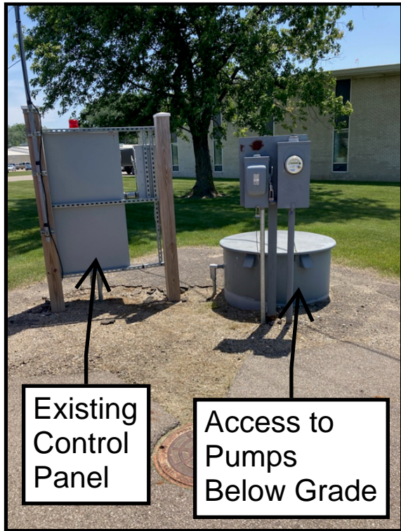
Liberty Street Existing Pump Station Condition
